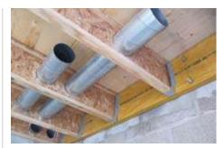
incoming air is blown past the outgoing air and is used to heat the incoming air. This has the effect of saving over 90% of the heat that, due to uncontrolled ventilation and draughts, would be lost in a more 'conventional' house.
