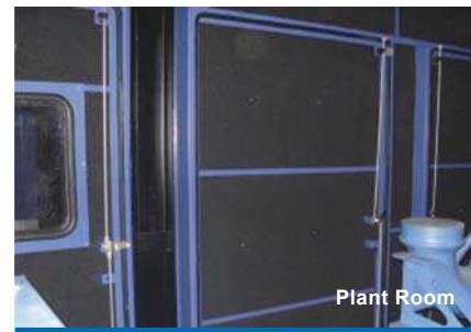
Insulating Ductwork Externally
