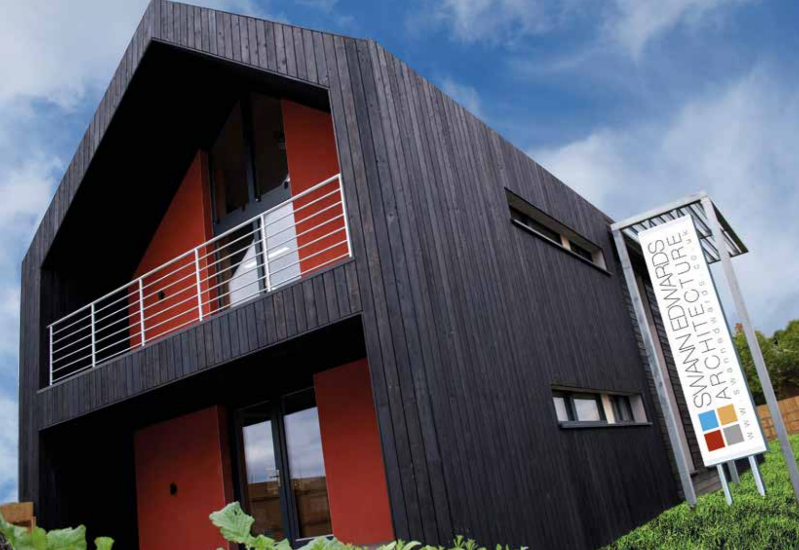
SWANN EDWARDS PASSIVHAUS OFFICE
