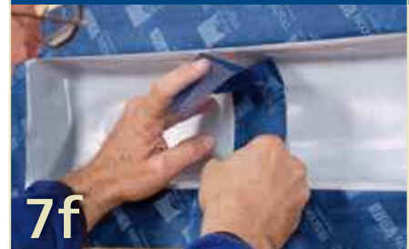
Enlarging: Taping over the overlaps
