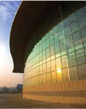
Solar control glazing to reduce the risk of over-heating
