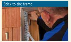
Begin to carry out the sticking in the corner area. First position approx. 2 cm of the tape on the horizontal part of the frame and stick the adhesive strip to the frame. Guide the tape around the frame corner and stick the tape to the vertical part of the frame. Gradually remove the backing paper while doing so.
