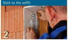
Gradually remove the second (wide) backing paper strip from the smooth membrane side. Begin to carry out the sticking to the soffit in the corner area. Stick the excess tape to the adjacent soffit side. Stick the tape into the next corner area. Stick the excess tape to the adjacent soffit side.
