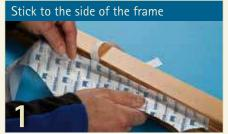
Remove the narrow backing paper strip, position it on the side of the frame flush with the frame edge and then gradually stick in place. The printed side of the tape must be facing upwards here.
