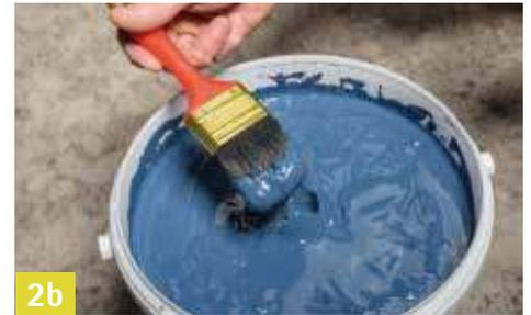
tected during spraying, these can be covered over with pro clima WYFLEXA fleece. To do this, paint AEROSANA VISCON onto a piece of fleece, apply the fleece to the defect and spray over it.
