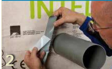
Fold the tape in the middle and remove the first release paper.
