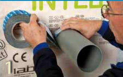
Roll out the tape to the required length and cut to size.
