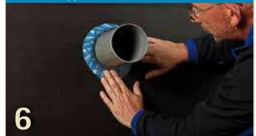
EXTLOSEAL MAGOV also provides secure joining of penetrations outdoors, e.g. through wall lining membranes, sarking membrane and roof lining membrane.
