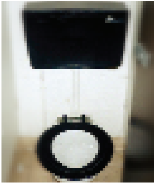
Old toilets before replacement
